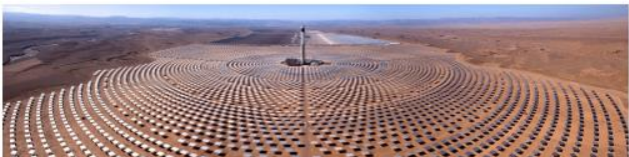
Morocco solar park - the project is one of the largest concentrated solar plants in the world. (ECOYZ, 2018)
